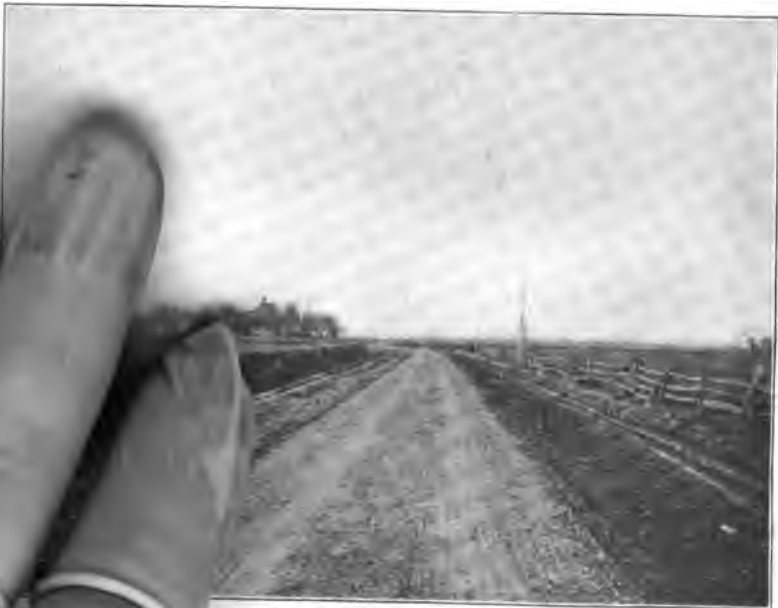
Neshanic road, Somerset Co., after improvement.
